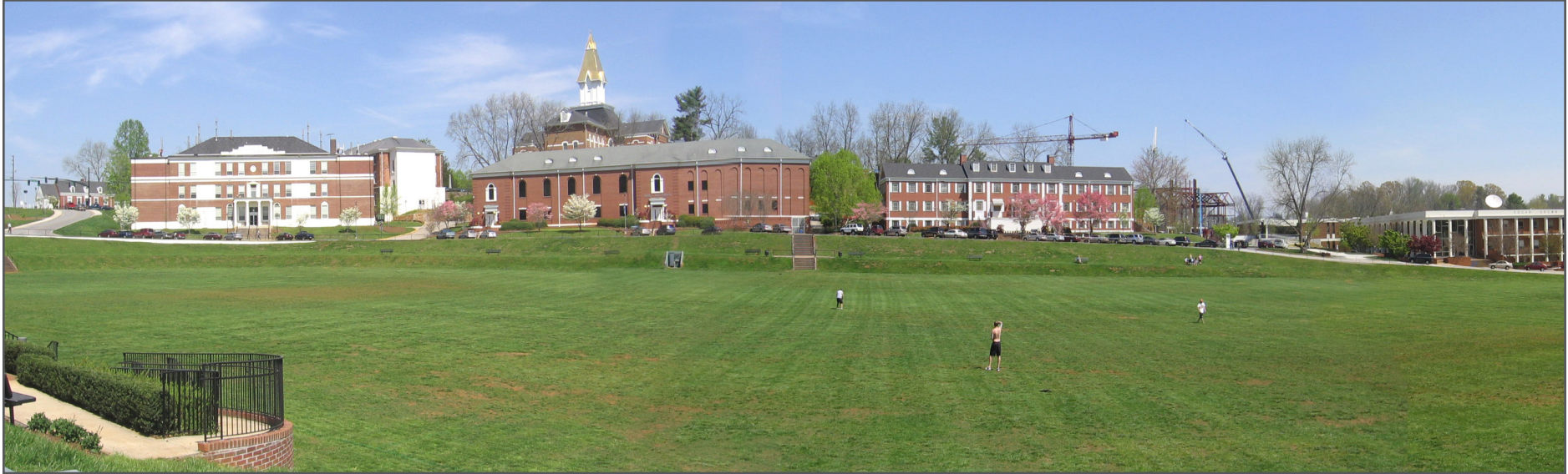
VIEW LOOKING ACROSS THE DRILL FIELD TO ACADEMIC BUILDINGS TO THE NORTH
